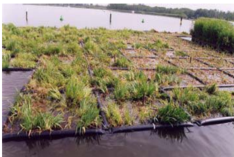
Figure 2. Floating wetland created by joining buoyant sub-units to create a floating frame to support plant growth (“Eco-Islands” by A.G.A. Group).
